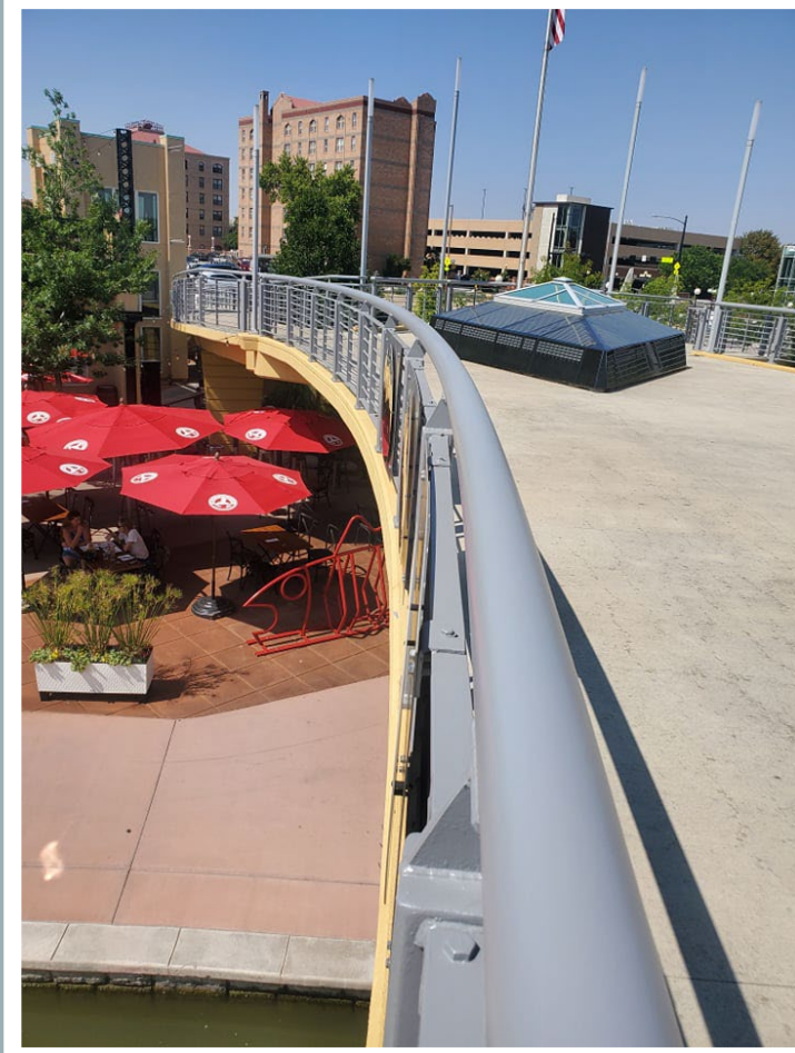
Veterans' Bridge Repair
