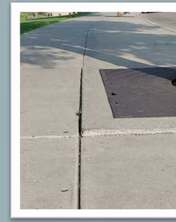
Walking Surface Leveling
