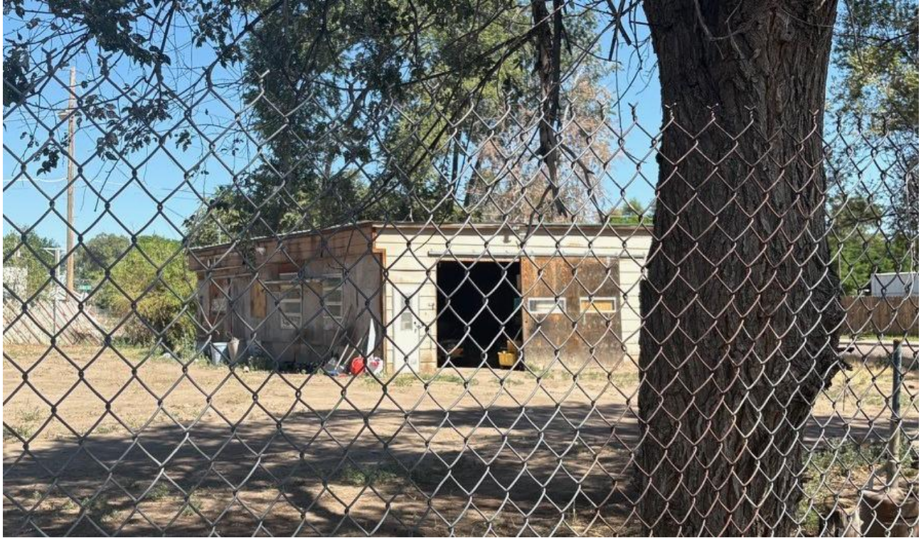
Existing structure, as seen from California St.
