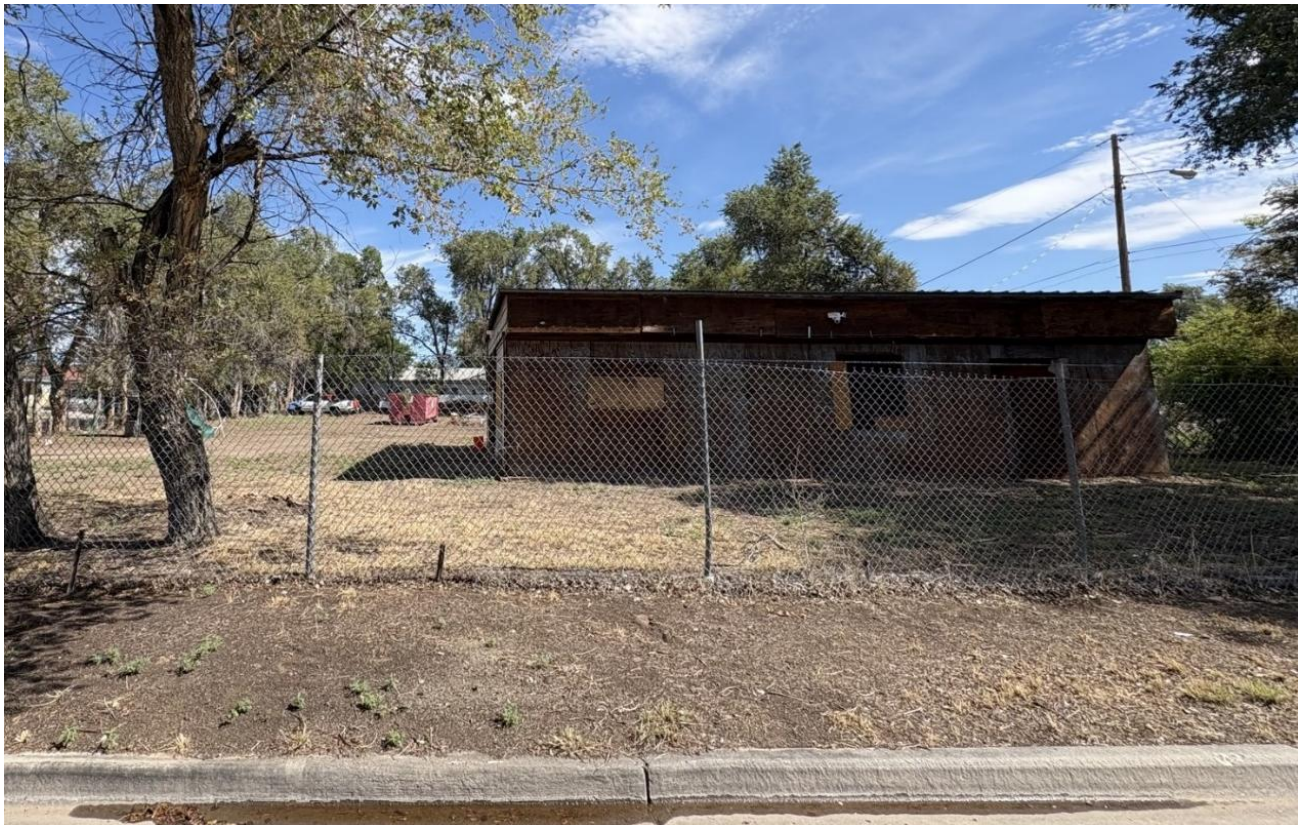
Existing structure, as seen from Nevada Ave.
