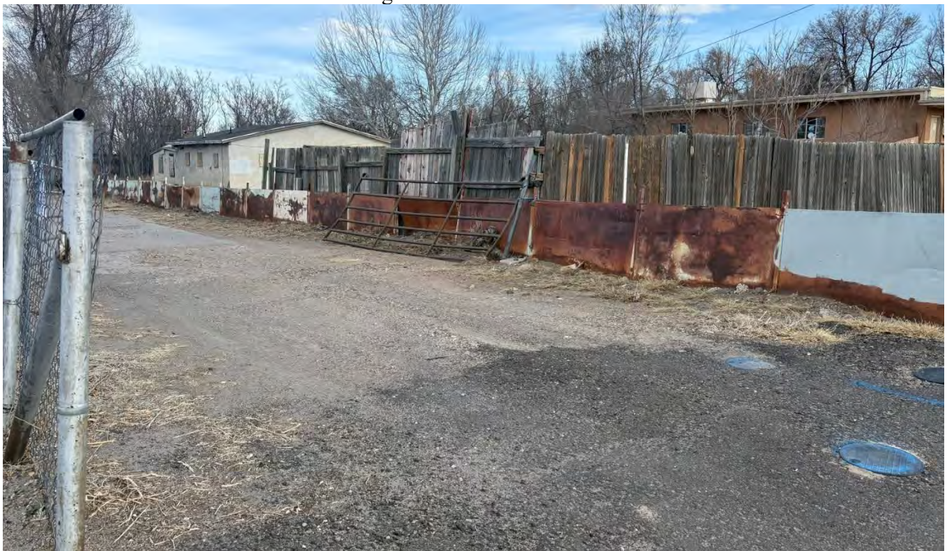
Beginning of Parcel A— closest to S Prairie Ave
