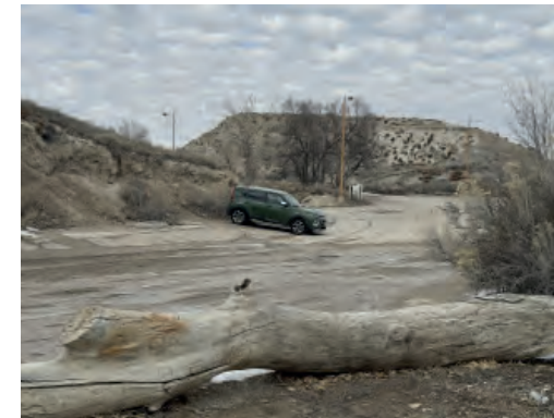
Parking lot drainage issues at Nature Center
