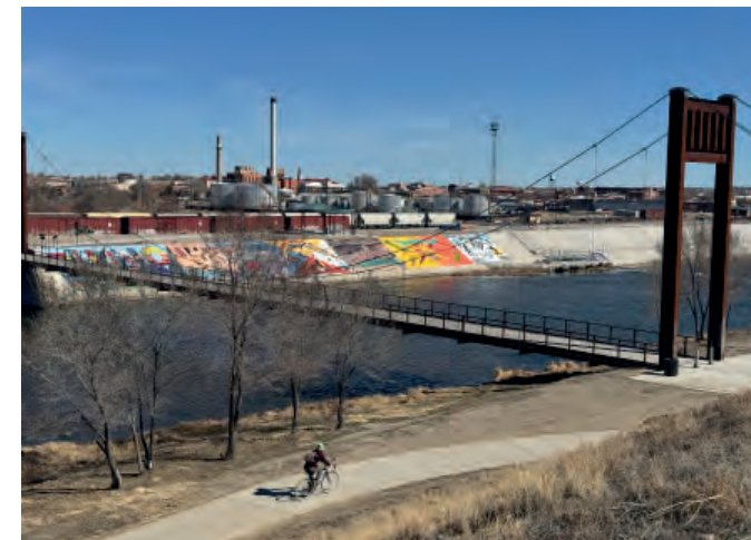
Trail in central corridor near Charles Lee bridge
