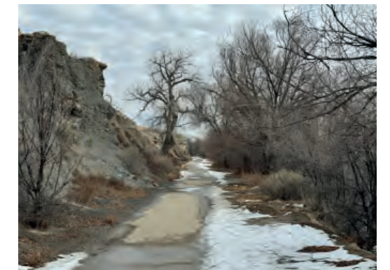
Erosion and maintenance needed for safety
