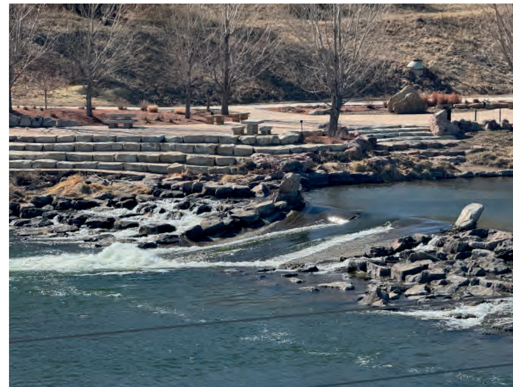
Drop Structure at Whitewater Park
