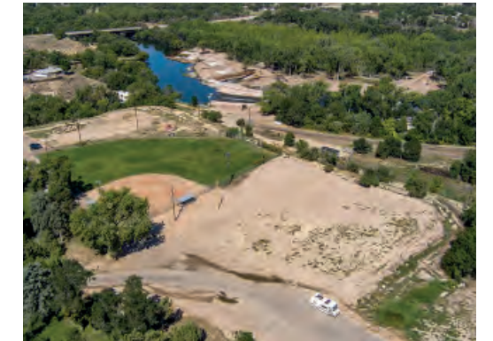
North edge of City Park is underutilized
