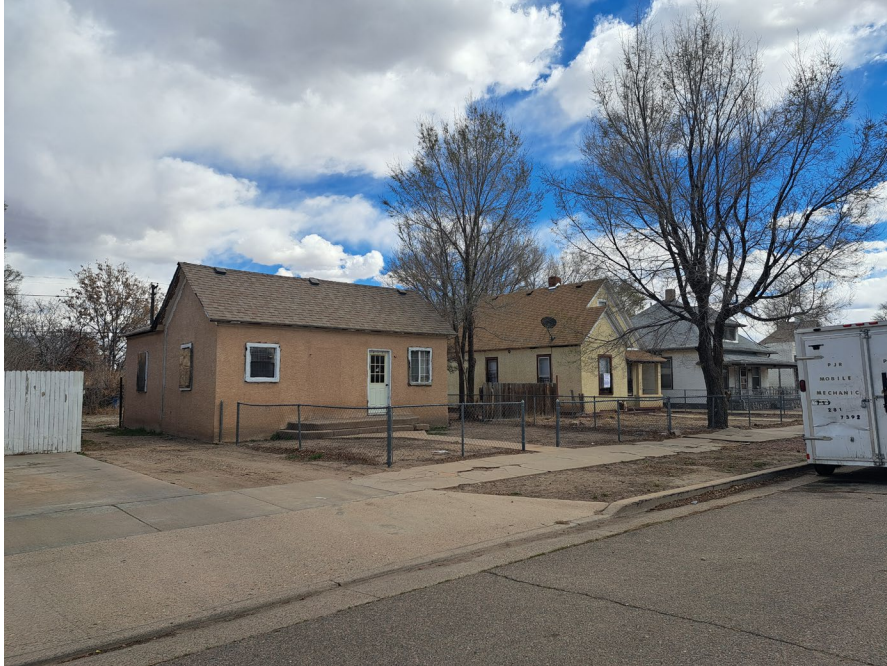
Overview of what used to be listed as 1328-26 Cypress St.
