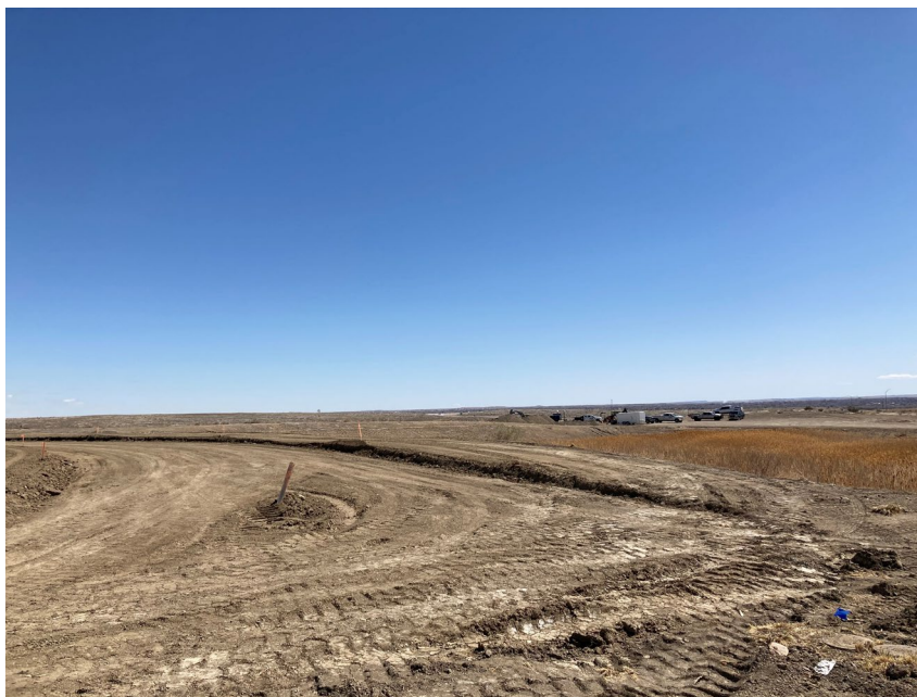
View of Residences at Villa Bella site looking northeast from Rawlings Blvd.
