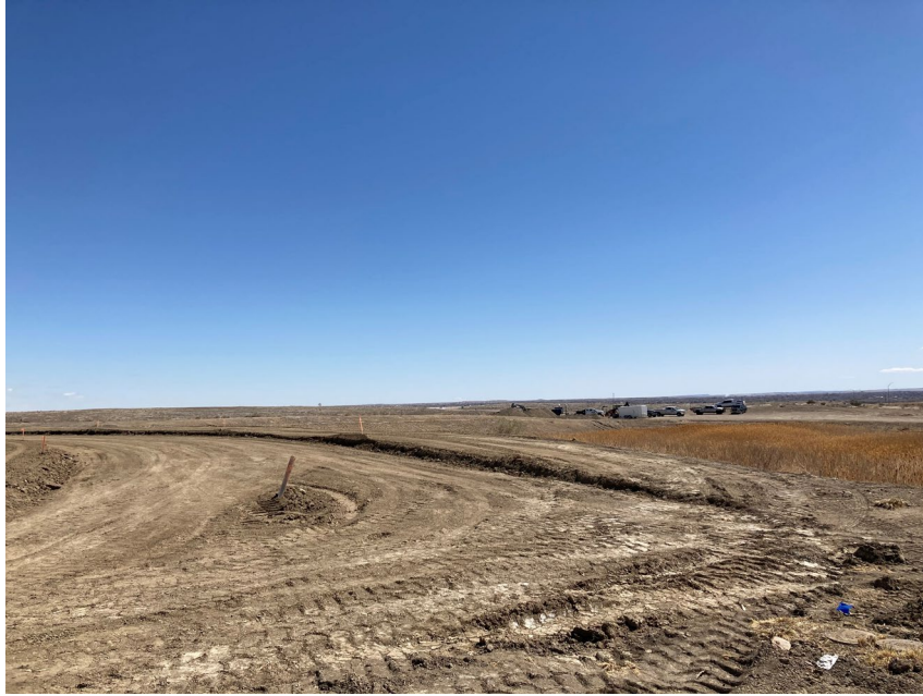
View of Residences at Villa Bella site looking northeast from Rawlings Blvd.
