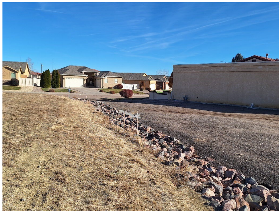
View of site looking west, drainage swale in foreground
