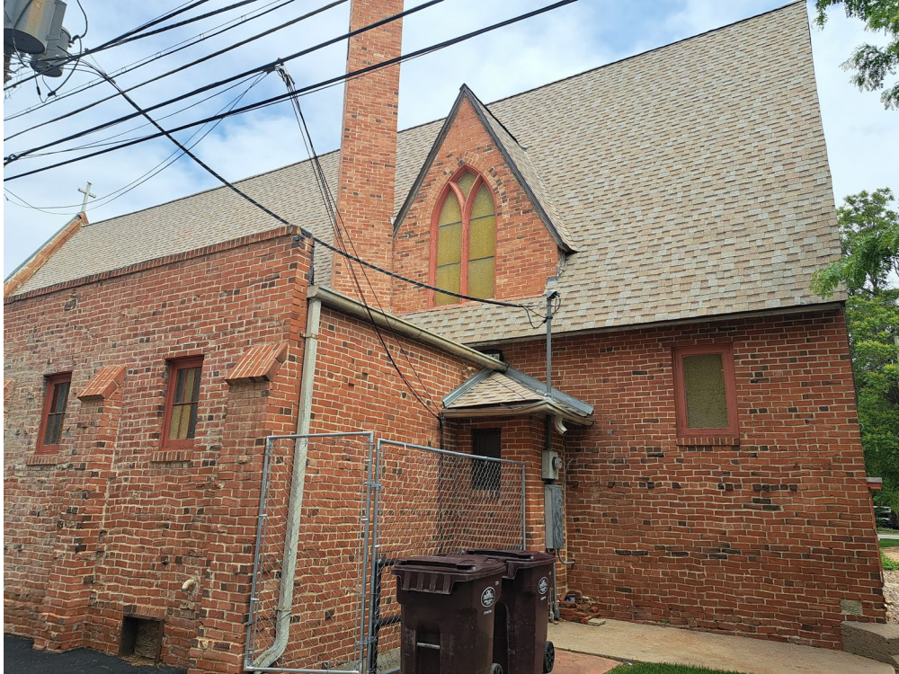
View of the chapel and rear corner
