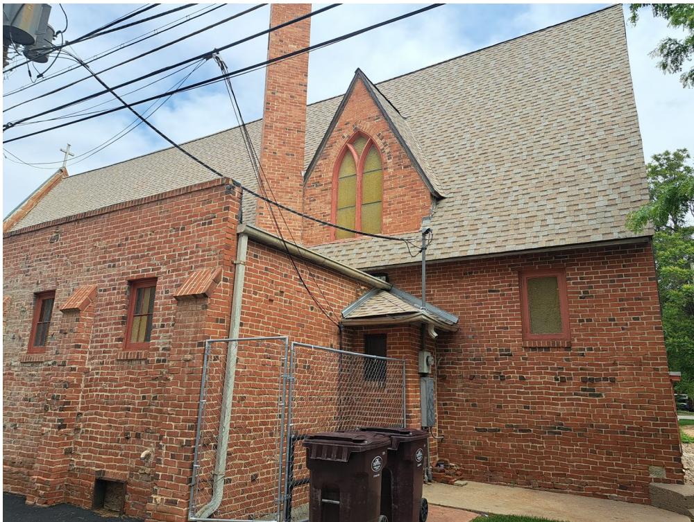
View of the chapel and rear corner
