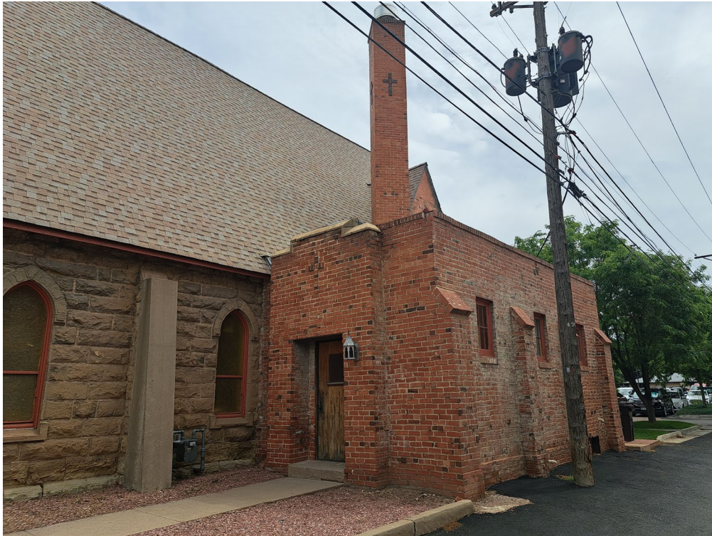
Overview of the small chapel.
