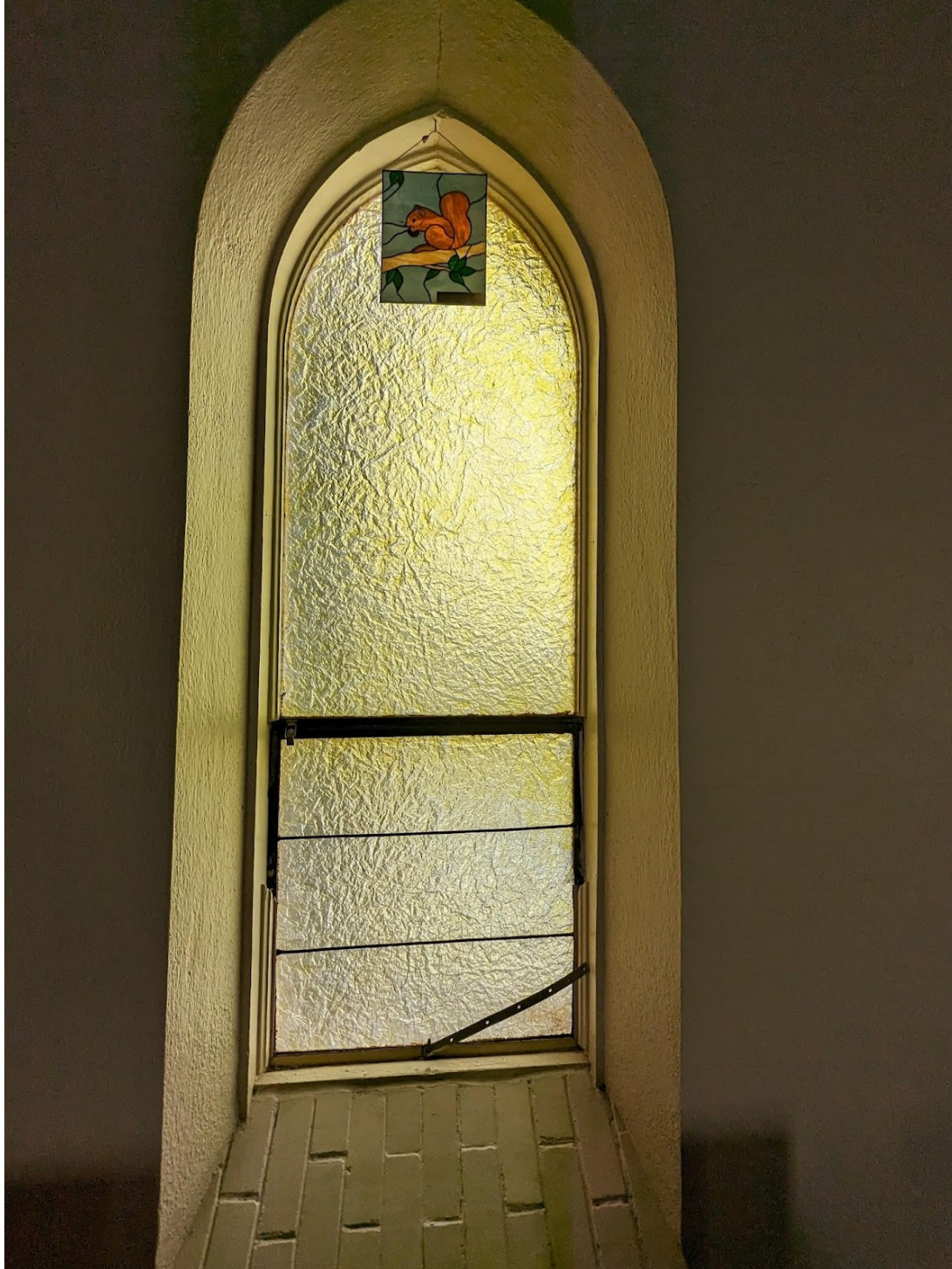
One of the sanctuary windows. The metal frames once had stained glass windows and are currently glazed with amber fiberglass. The angular bar is to open or lock the hopper at the bottom of the window.
