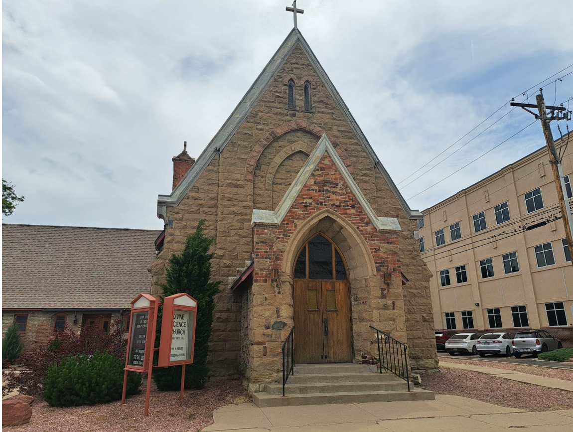
Overview from front façade showing parapeted
