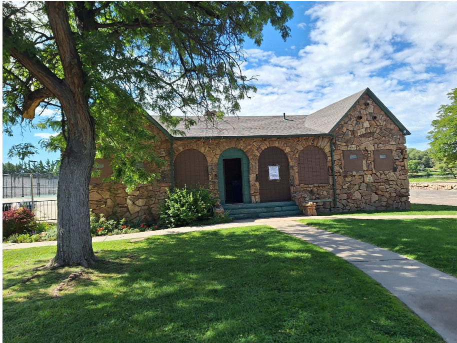
Overview from front façade looking south
