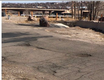
Potholes and Alligator Cracking
