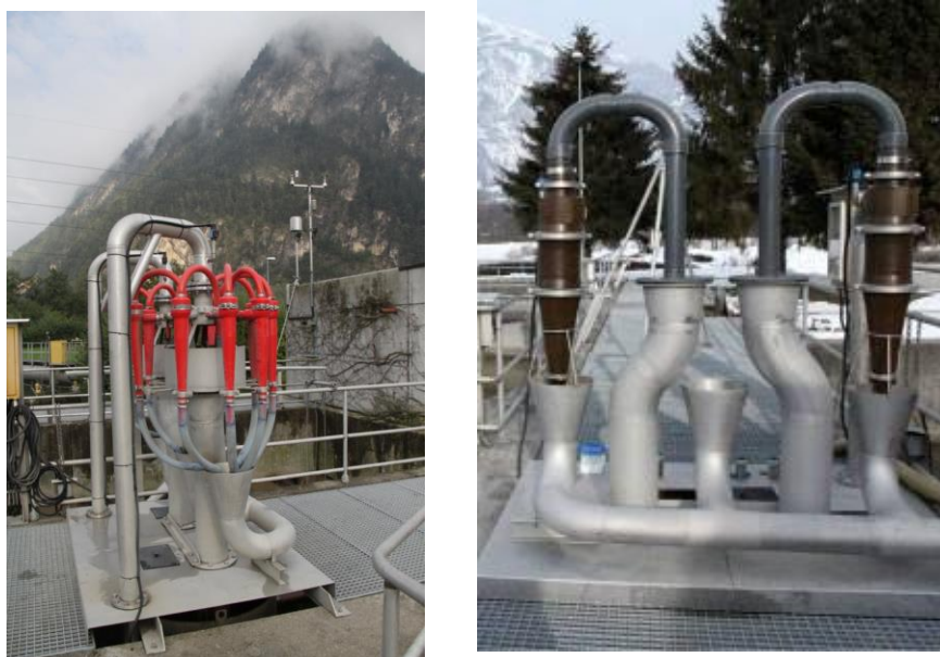
Figure 12-2. Photos of full-scale hydrocyclones
