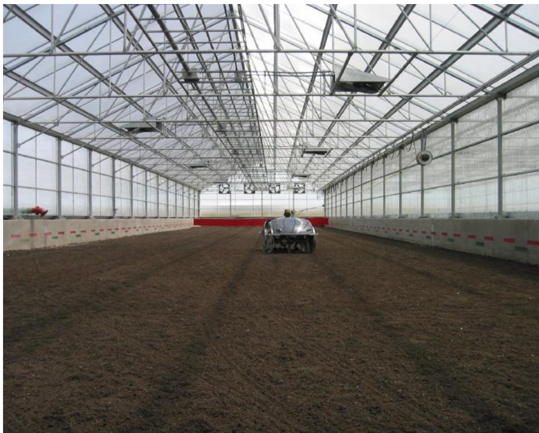
Figure 23. Photograph of a Solar Dryer with Electric Mole (Figure Courtesy of Parkson)
