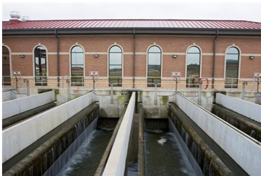
Figure 12-4. Example Severn Trent Denite® filters
