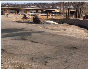
Potholes and Alligator Cracking
