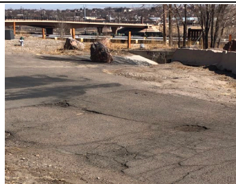
Potholes and Alligator Cracking
