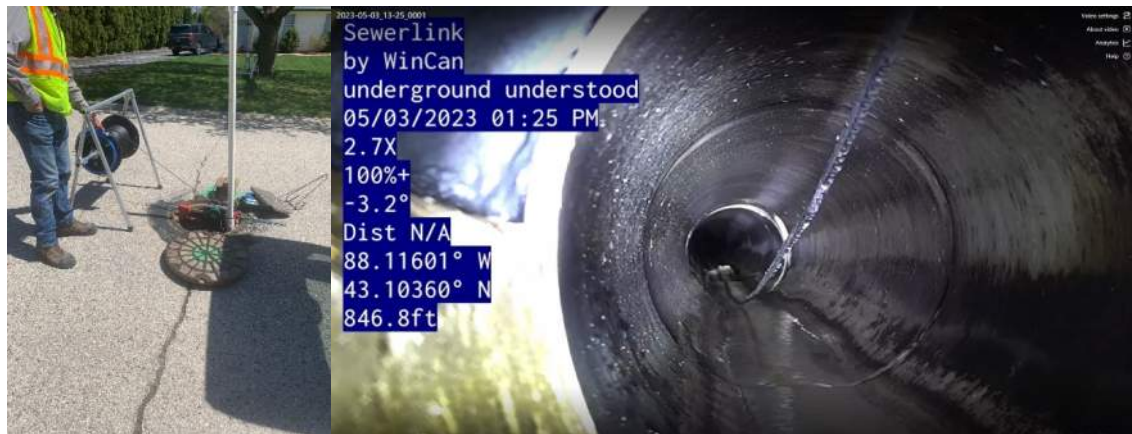
Figure 5. Street View of manhole and interior pipe view.
