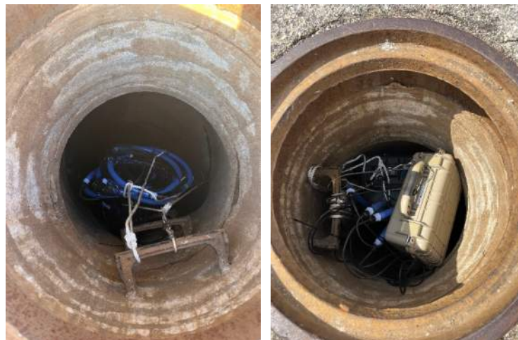
Figure 6. DTS cable secured and installed within manhole.
