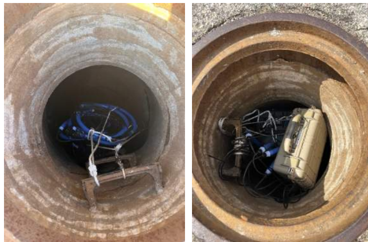
Figure 6. DTS cable secured and installed within manhole.
