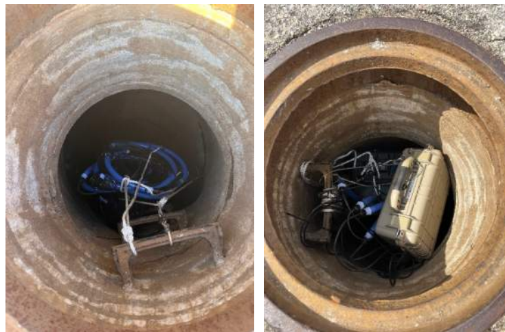
Figure 6. DTS cable secured and installed within manhole.
