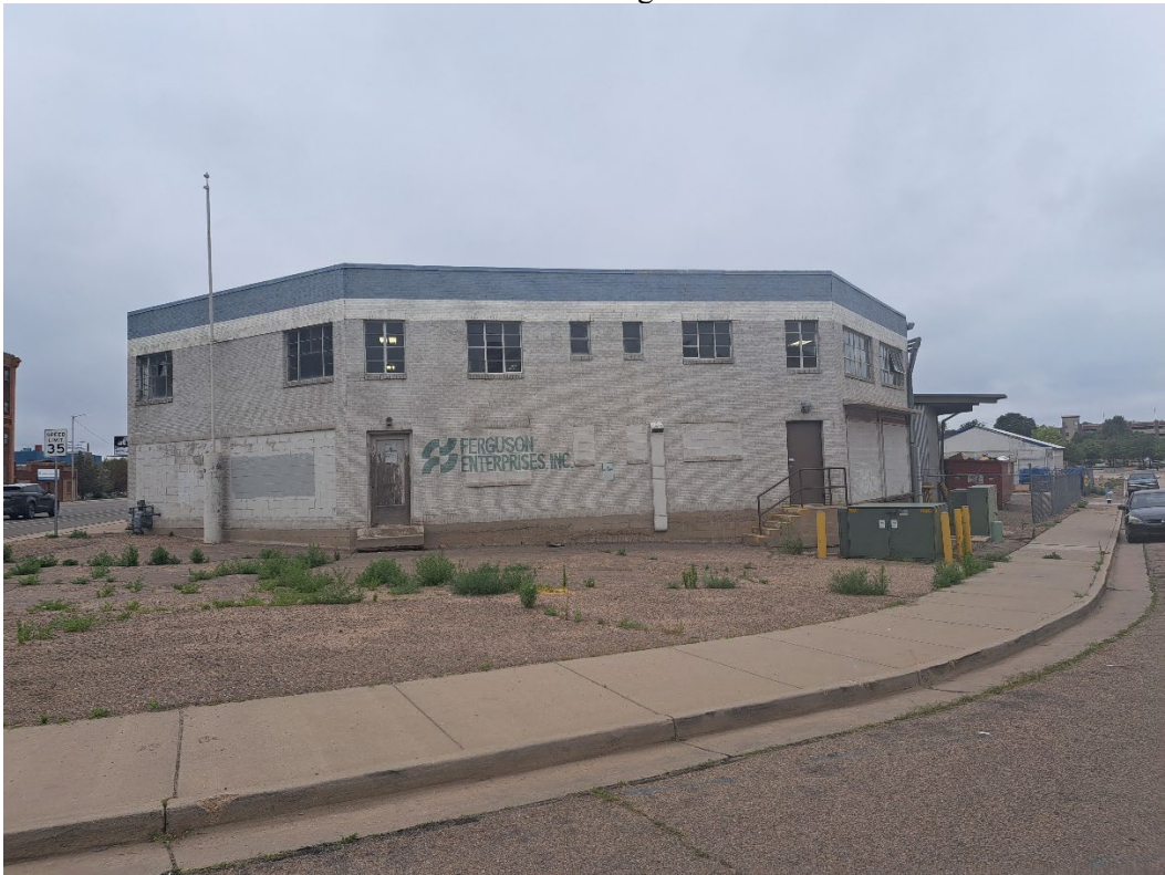
D Site Photographs. View the main Ferguson’s building along Santa Fe Dr.
