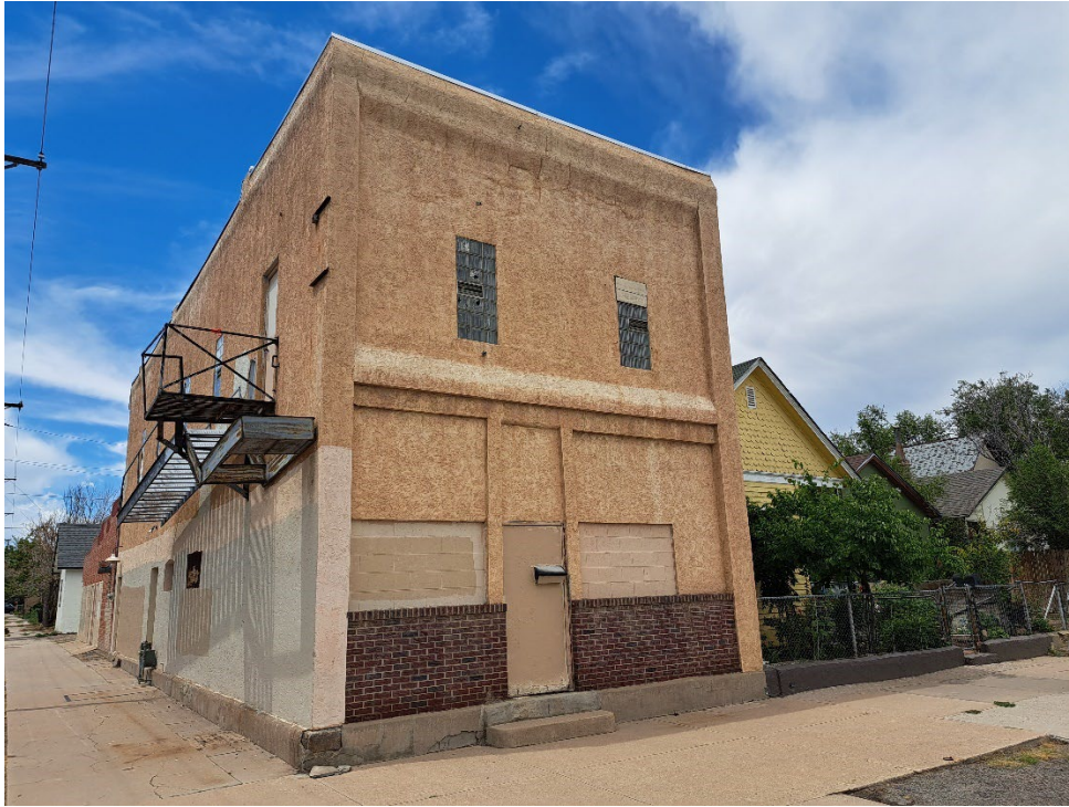
E2. Overview of 945 E. Routt Ave
