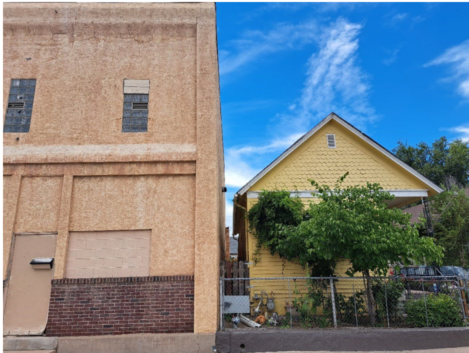
E8. Overview of the northern property line looking west.
