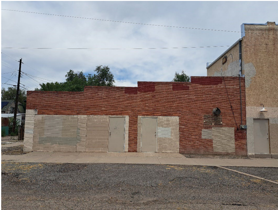
E3. Overview of the later rear 1 story addition.
