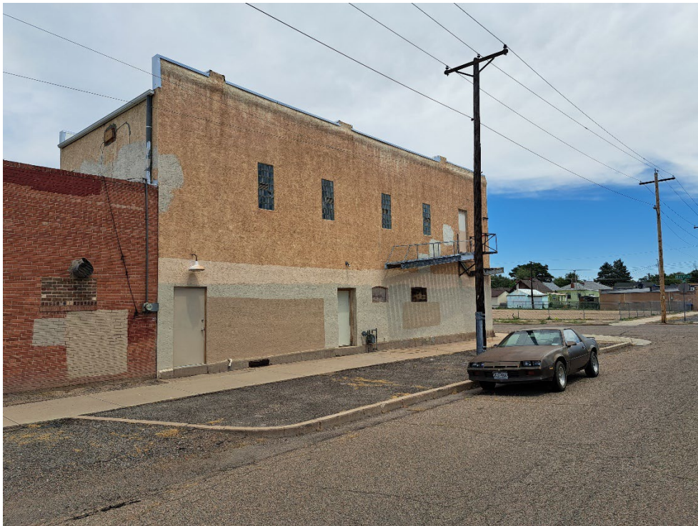
E4. Overview of the building from Summit Avenue.
