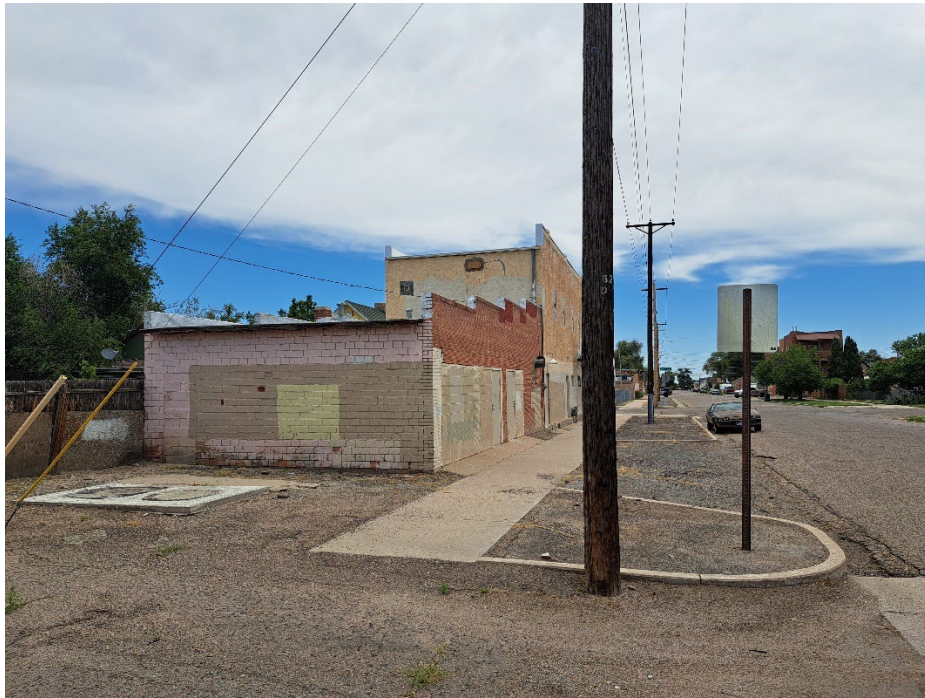
E6. Overview of the rear of the property.
