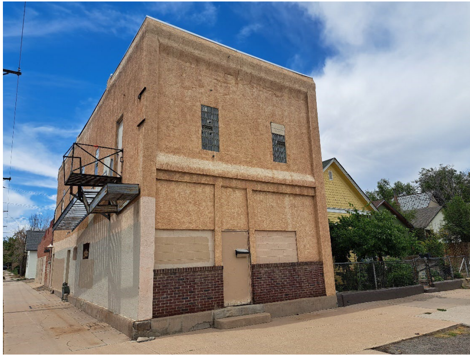
E2. Overview of 945 E. Routt Ave
