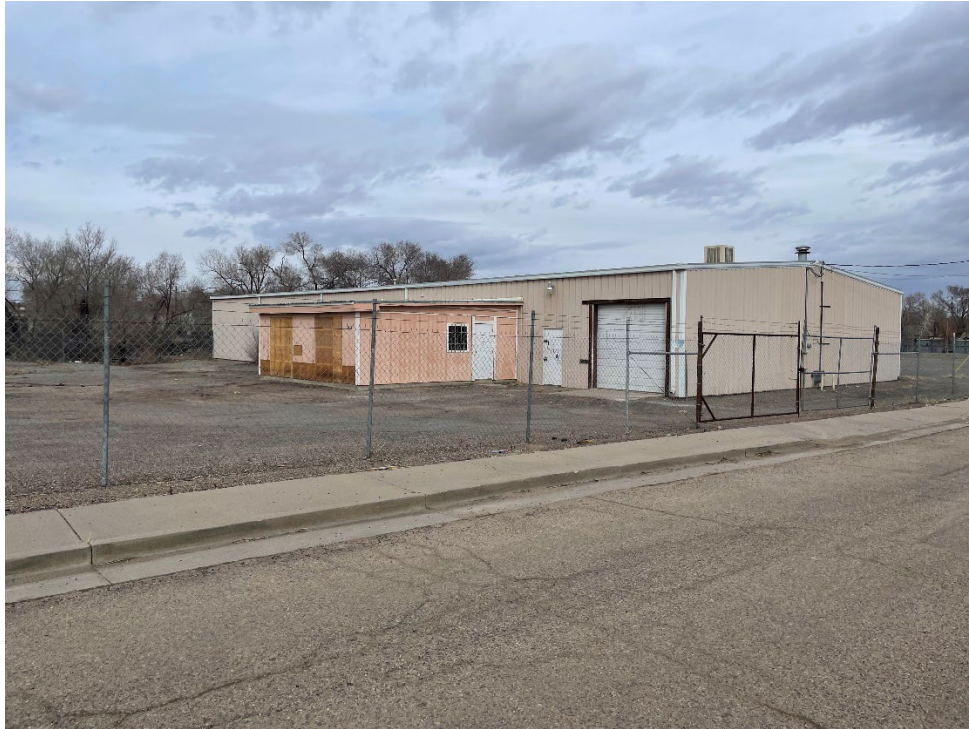
D. 2511 E. 4 th Street looking north from Dry Creek Rd.
