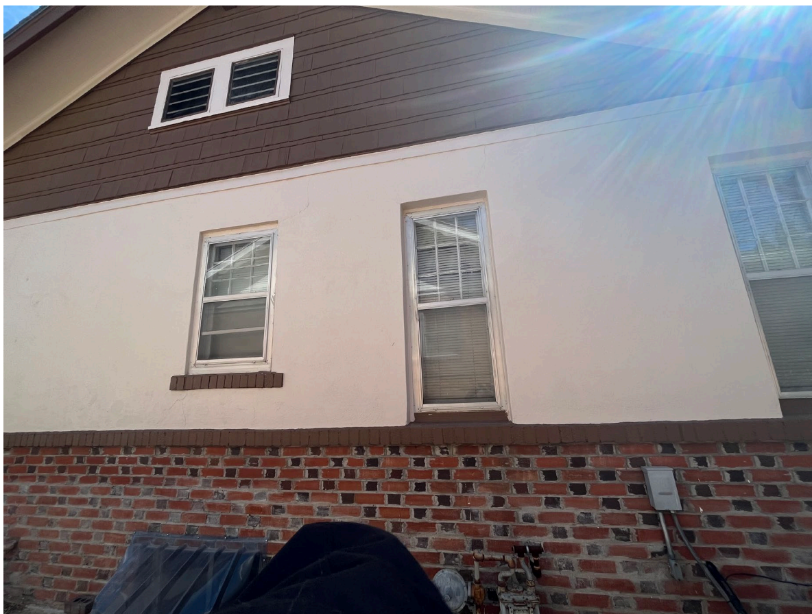
Eastern façade close up
