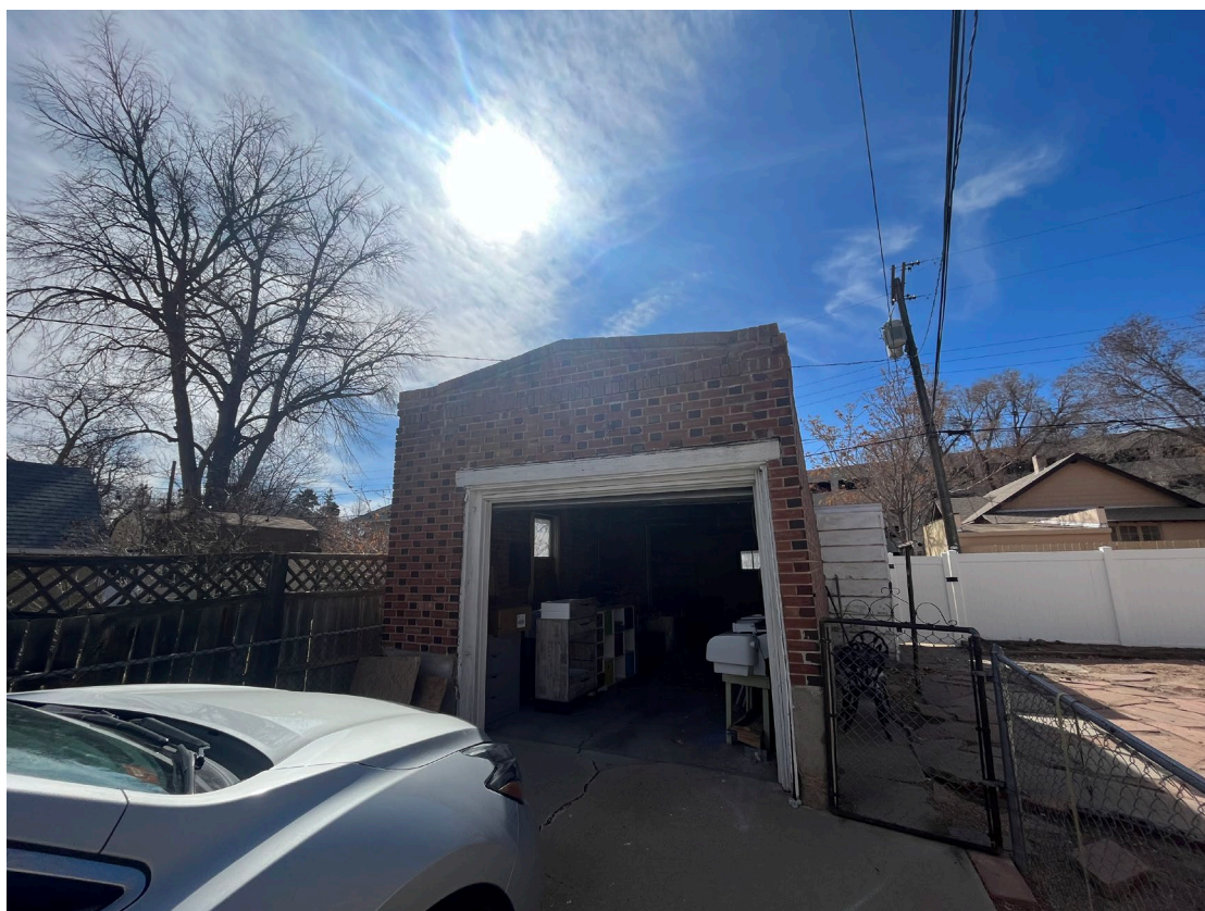
View of garage looking south.
