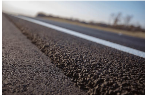
Thin Lift Overlay
