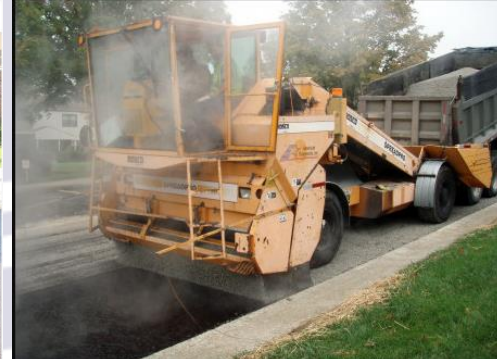
Cape Seal (Chip + Slurry)
