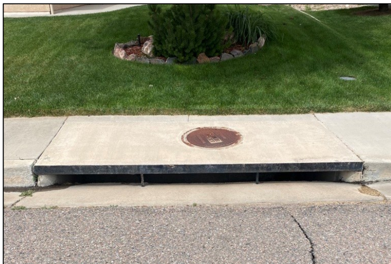
Photograph 8-2. Curb opening inlet in City of Pueblo.
