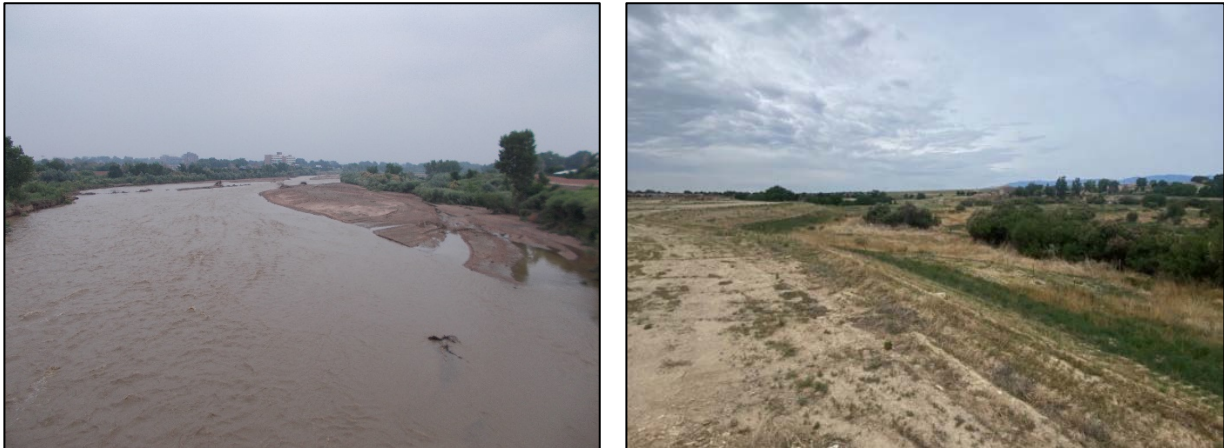
Photograph 4-1. Fountain Creek (left photo) is a major drainage that runs through the City of Pueblo and is designated as a FEMA Special Flood Hazard Area (SFHA). Goodnight Arroyo (right photo) is a smaller channel with intermittent flow which is also located within the City of Pueblo and is mapped as a SFHA. These examples demonstrate the wide range in channel types that are mapped as regulatory floodplains by FEMA.
