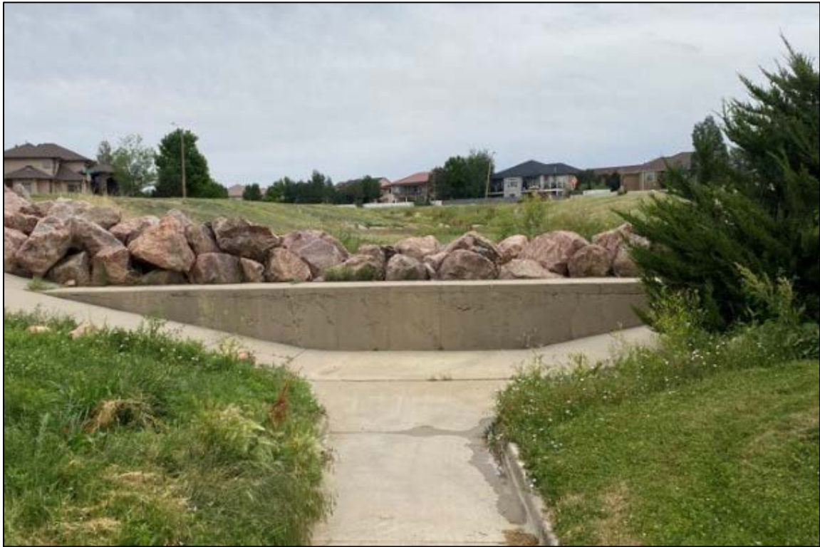
Photograph 11-5. A series of rock riffles is generally a preferred approach for achieving grade control in a channel as opposed to a vertical structure such as the one shown in this photo. Where used, vertical grade control structures should have a drop of less than 3 feet.
