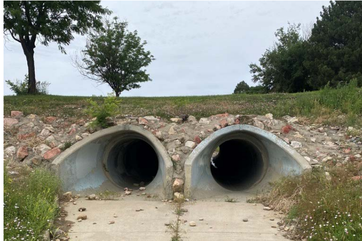
Photo 12-1. A twin-barrel culvert with flared-end sections is shown with a grouted rock headwall.
