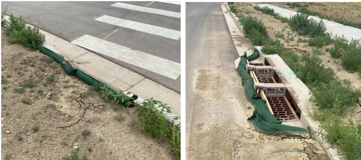
Photo 15-1. Examples of sediment control and inlet protection during construction activities
