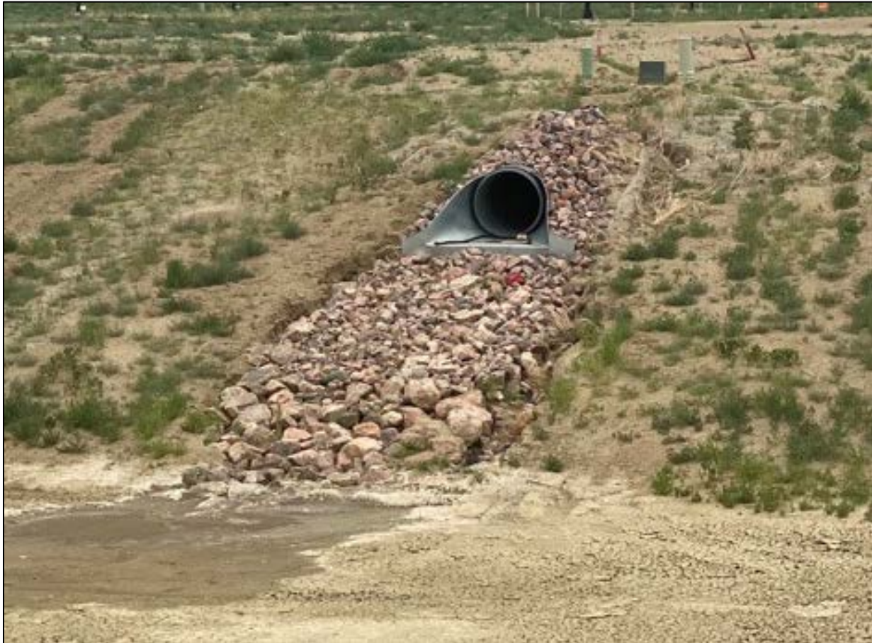
Photograph 9-4. Riprap protection at storm drain outlet
