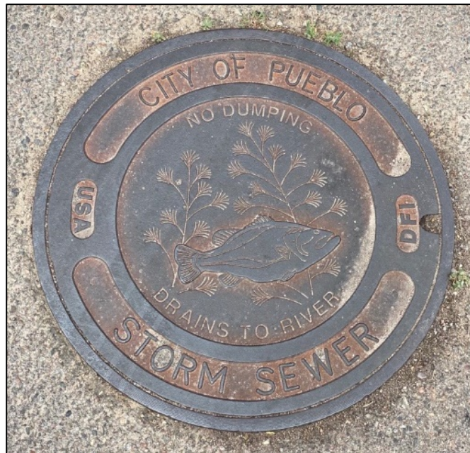
Photograph 9-3. Manhole covers for the storm drain system in the City of Pueblo alert the public to “No Dumping” because of the system’s discharge into receiving streams.
