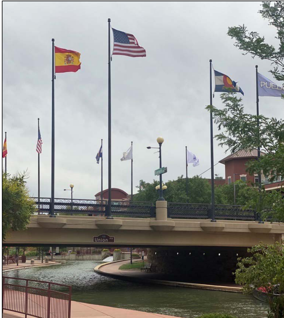
Picture 12-2. Bridge on Union Avenue crossing Pueblo's Historic Arkansas Riverwalk.
