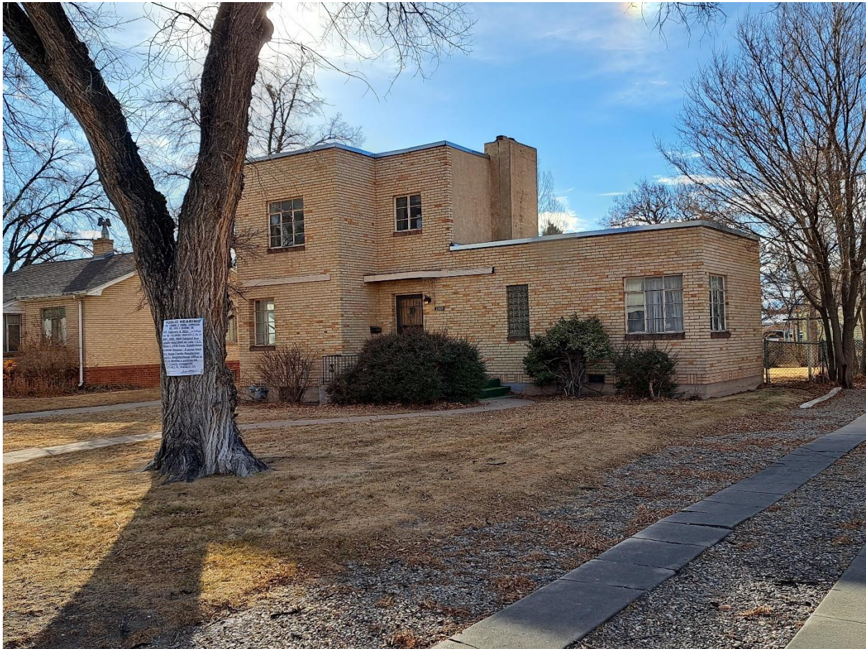
D. Southern building (2009 Oakland Ave) being removed for the parking lot
