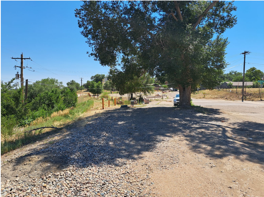
Site overview looking southeast
