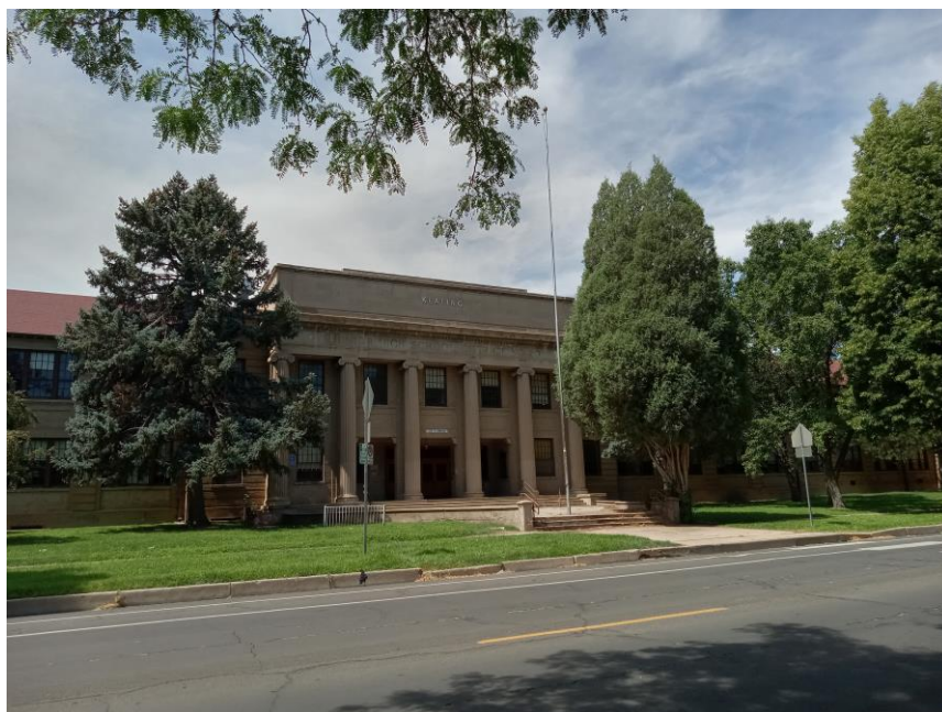
Looking Southwest from Orman Ave.
