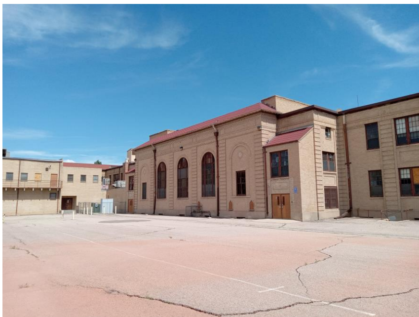
Overview of the theatre and rear access
